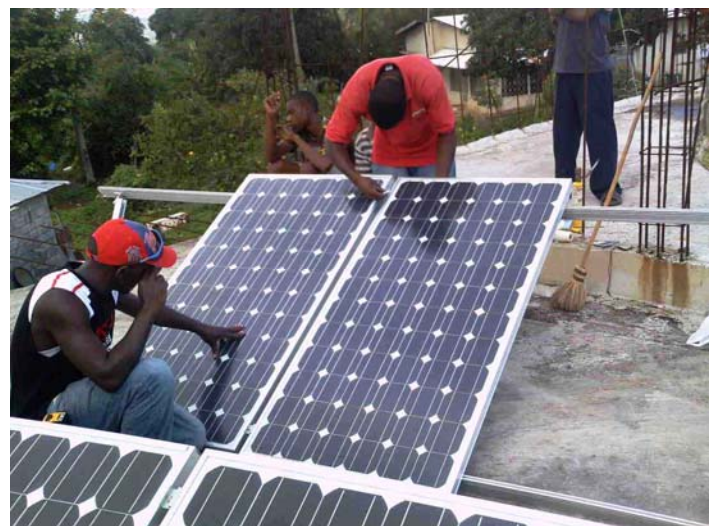
Solar panels being installed at the Jeffrey Town Community Centre
